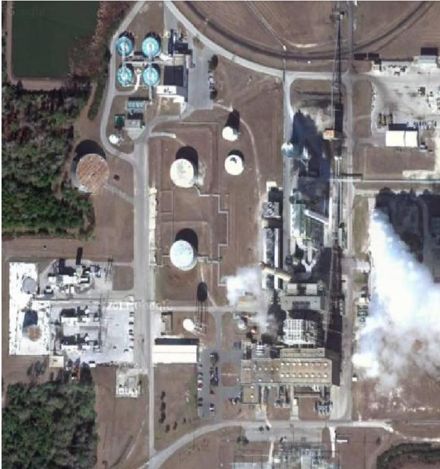
Deerhaven Power Plant north of Gainesville, Florida. Toxic vapors billow constantly 24/7 from this coal-fired power plant north of Gainesville, Florida, adding a constant mist of pollution to the air. Florida had 30 coal-fired generating units at 14 locations in 2005, with 11,382 megawatts (MW) of capacity -
