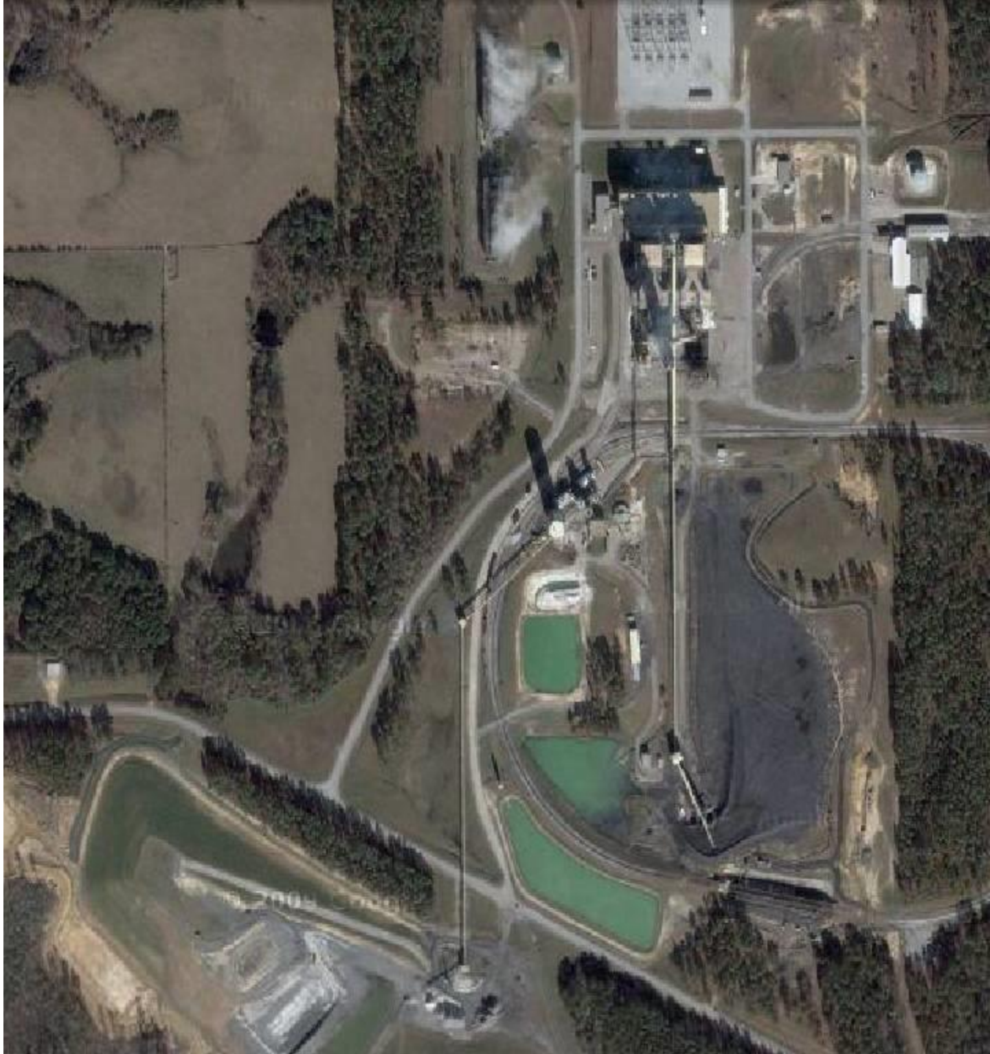
Morrow Generating Plant near Hattiesburg, Mississippi (Source: Google Maps )
